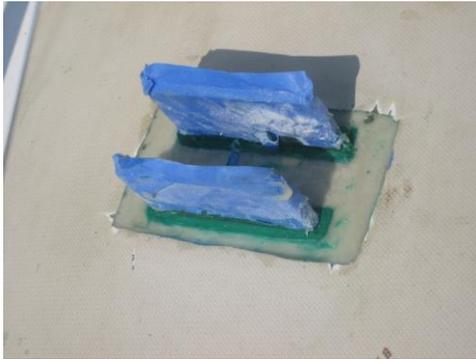
Before you remove the craft paper, do a rough grind of the surface of the epoxy be sure there are no really low spots.
