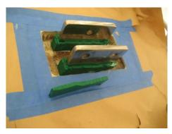
Buy a block of kid's modeling clay. Cut strips that are 1" high and  $\frac{1}{4}$ " to  $\frac{5}{8}$ " thick and carefully press them against the chain plates being careful that they go all the way to the lower surface and are at least as high as the top deck surface.
